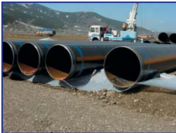
Borcoat bimodal PE pipe coating provides a three-layer system for steel pipeline. Borealis.
